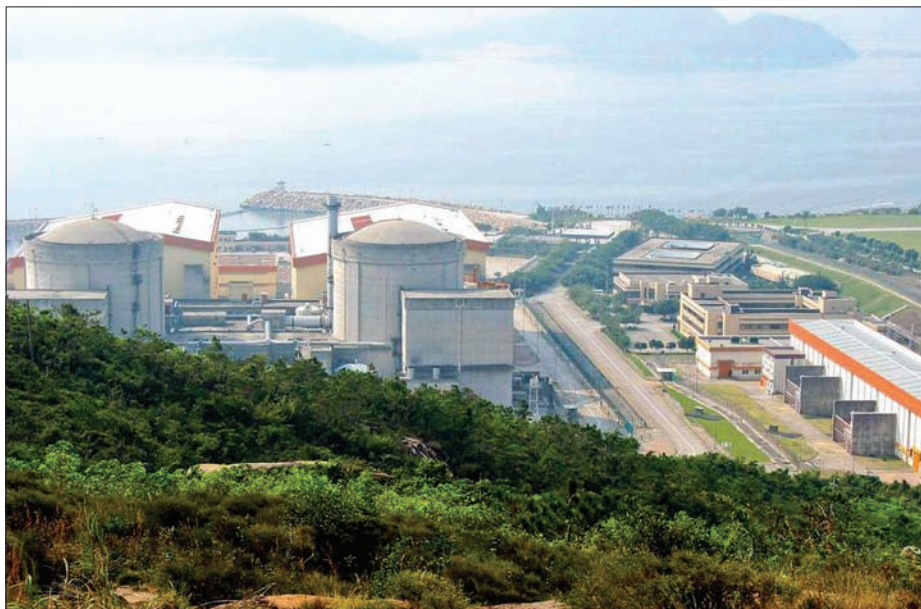
The nuclear power plant at Daya Bay. (Image credit: IHEP.)
