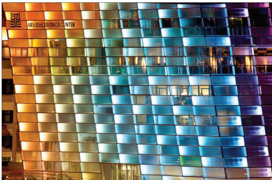
LED strips mounted behind the glass panes illuminate the façade of the Ars Electronica Centre in Linz. (Image credit: Nicolas Ferrando, Lois Lammerhuber.)
